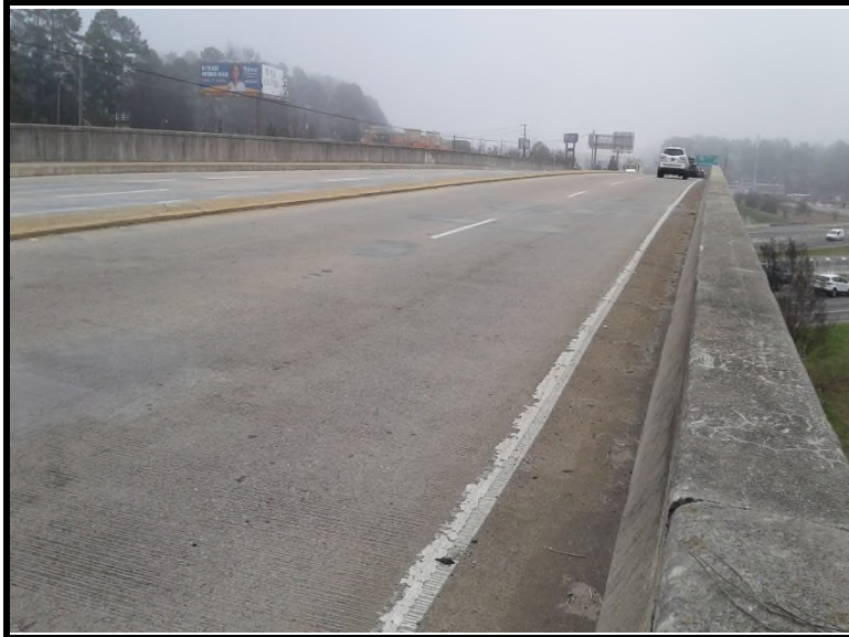
1 View of the Bush River Road Bridge over I-26.
